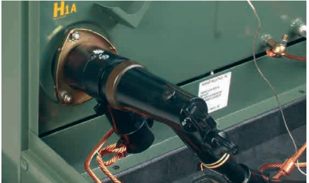
Single-bushing transformer To add surge protection to a single-bushing transformer, use a bushing arrester or an elbow arrester with a feed-through insert.
