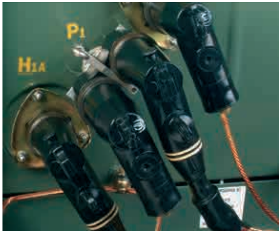
Two elbow arresters and a feed-through This approach uses elbow arresters only. (One of the elbow arresters may be mounted on the H1A bushing if operating procedures permit.)
