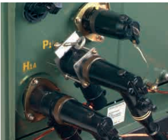
Bushing arrester and parking stand arrester* This approach is best for increasing operability and reducing transformer overcrowding.
