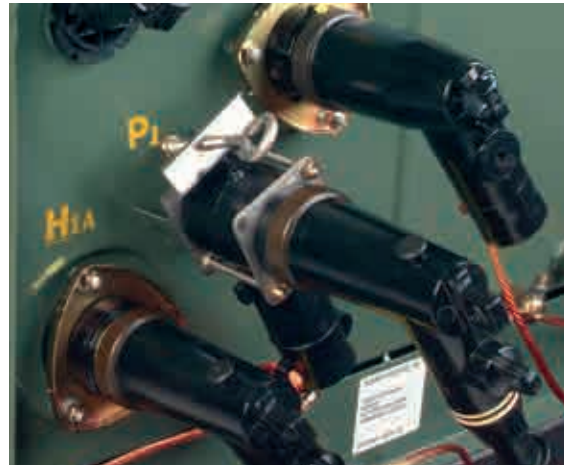
Elbow arrester and parking stand arrester This approach can reduce overcrowding by eliminating the feed-through device. This is desirable in a mini-pad transformer.
